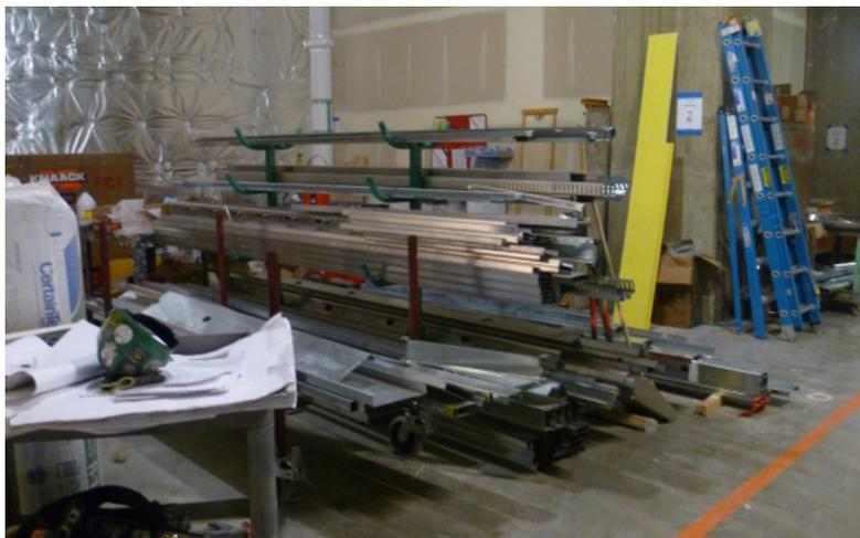
Figure 4. The pre-cut studs were stored in their intended locations.
